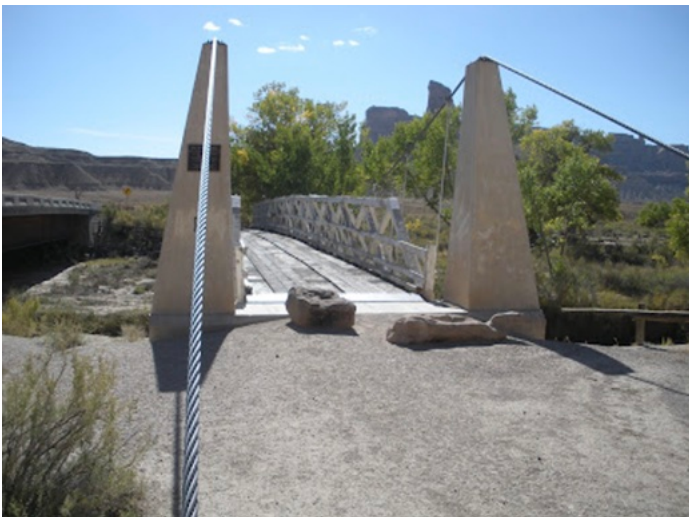
The “old” bridge crossing the San Rafael River in the middle of the Swell. It was infamous for moaning and groaning and sagging whenever a car slowly crept from one bank to the other. A new ugly, concrete bridge, seen to the left, was offered as a replacement.
